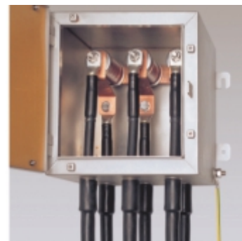
Link box installed with cross bonding cables
